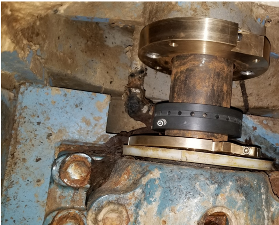
SEPCO SAS installed for a pulp and paper manufacturer
